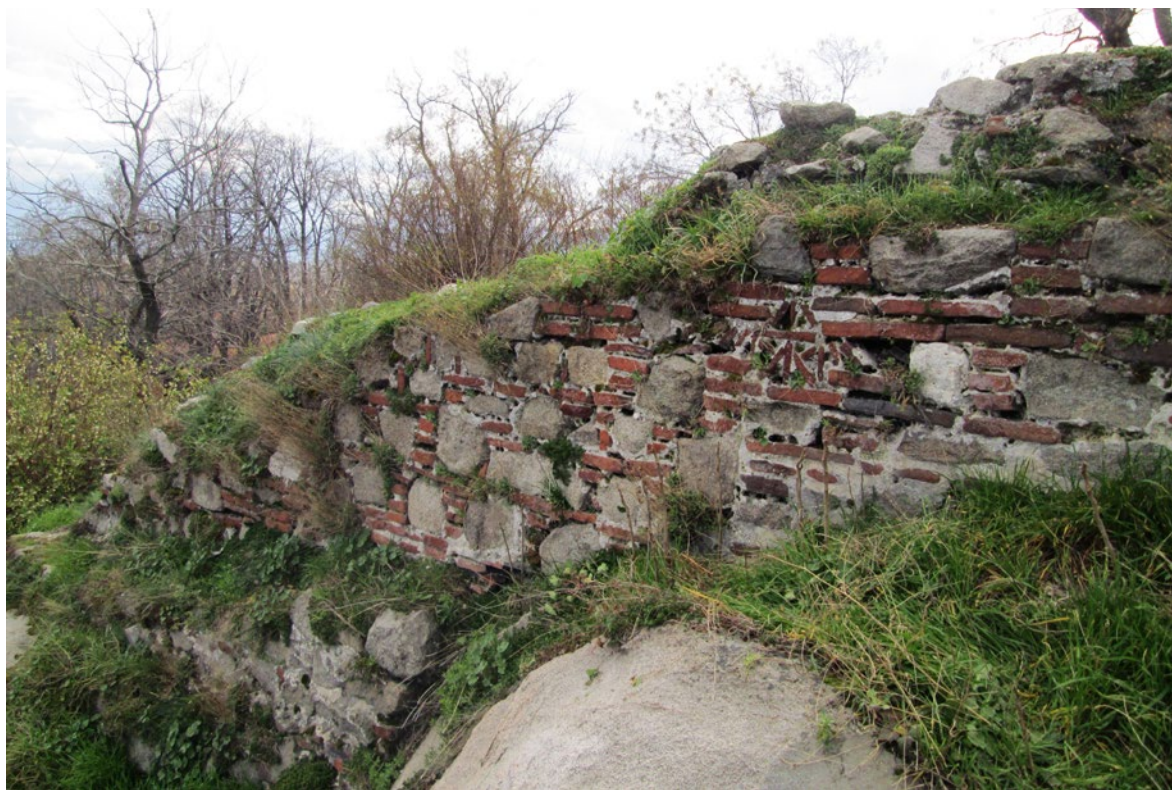
Fig. 8. Newly built route in the northern part of the eastern wall on Nebet Tepe, end of the 12 th – beginning of the 13 th c.
